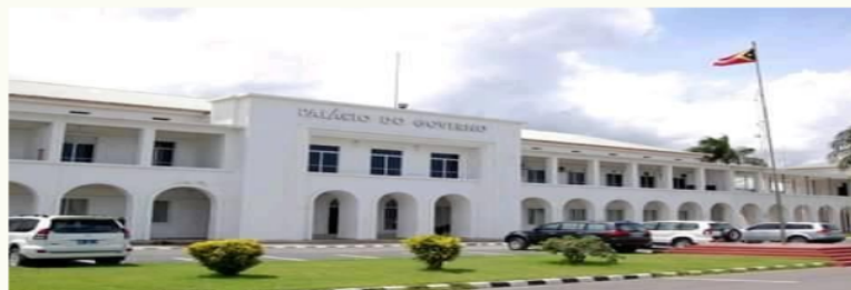
Picture 2 : Timor Leste Government Building 22
